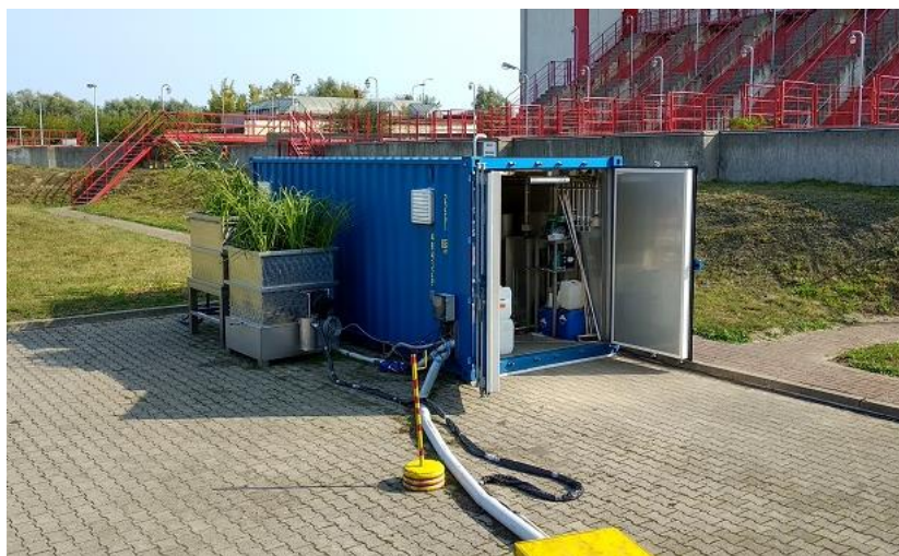
Fig. 2 View of the pilot plant located at the Wschód WWTP.
